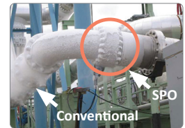
Cryogenic applications Leaking conventional flanges vs. leakfree Vector SPO® Compact Flange.
